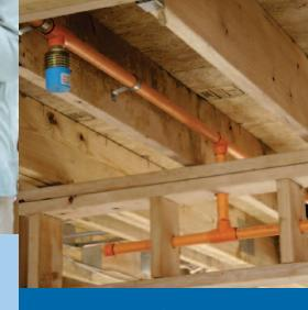
Sprinklers are linked by a network of CPVC piping hidden behind walls and ceilings in finished areas.
